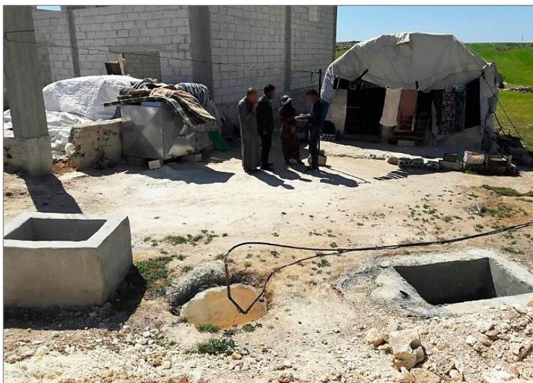
A newly installed biogas well.
