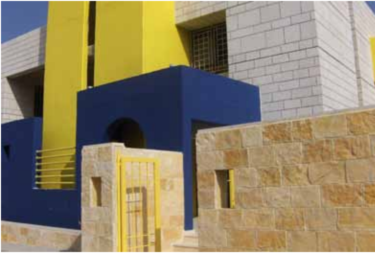
The Safer Children's Center in Palestine has 50% less power needs than similarly sized buildings nearby due to the use of green building techniques such as a grey water treatment system and low-cost sunshades.
